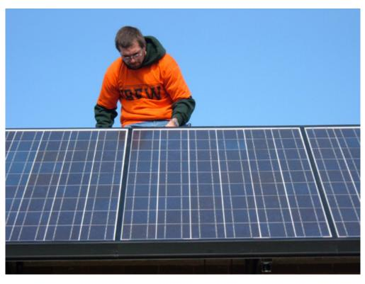
Jacob Grovogel puts the finishing trim on the tops of the panels. The 5-kilowatt solar-electric system is installed on the South wall of the Labor Temple.
